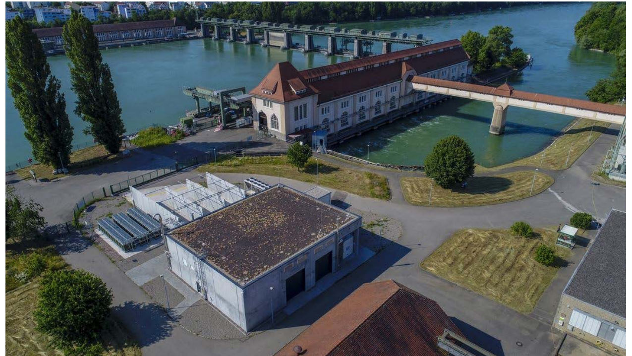
Southern Germany's largest plant for green hydrogen is being built at the Grenzach-Wyhlen site. https://www.enbw.com/company/press/enbw-starts-marketing-green-hydrogen.html
